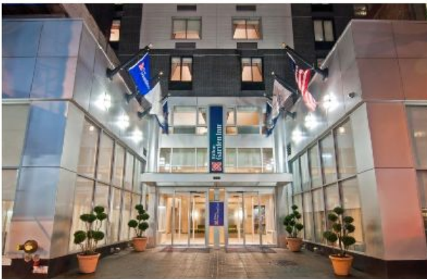
Entrance off 28 th Street
