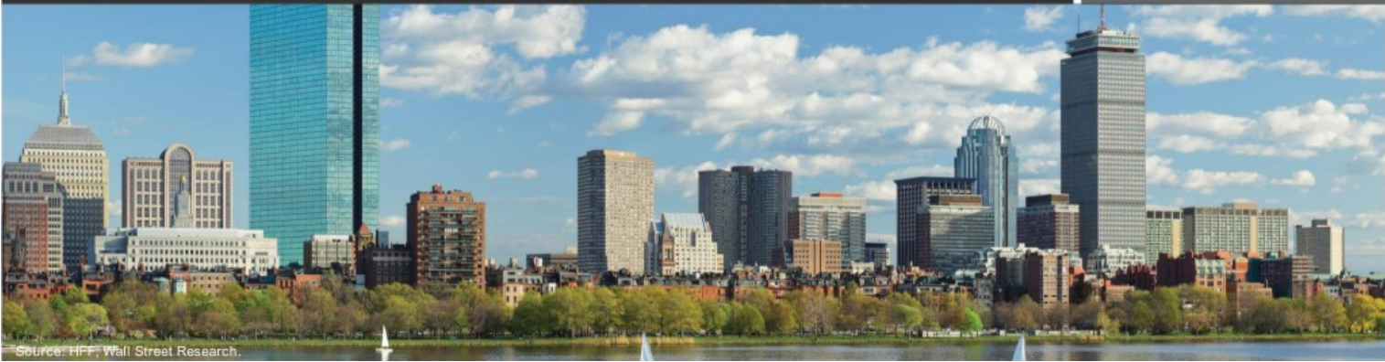
Source: HFF, Wall Street Research.
